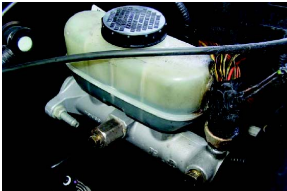
Another speed control deactivation switch in the early stages of fire beginning to burn the plastic brake fluid container
