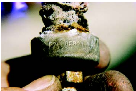
Remains of damaged switch found at scene
